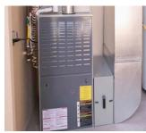
A furnace heats air and uses a blower motor and air ducts to distribute warm air throughout the house.
