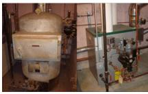
A boiler heats water to provide hot water or steam for heating that is distributed through a series of pipes.
